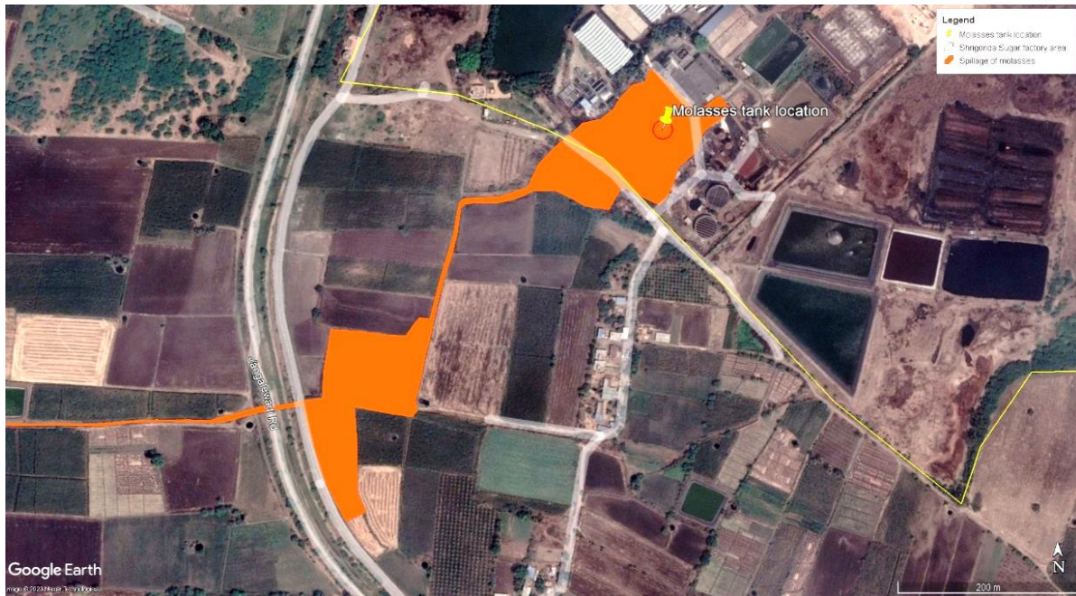
Figure 3.2: Image showing spillage of molasses outside factory premises
