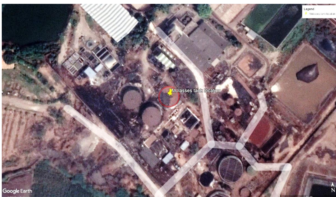
Figure 2.1: The place (tank location) of accident
