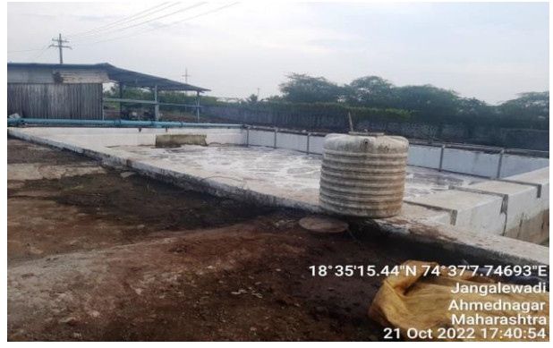
Photograph-2: ASP of sugar unit ETP under stabilization process.
