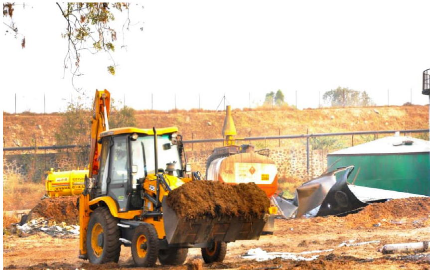
Figure 2.3: Removal of contaminated soil
