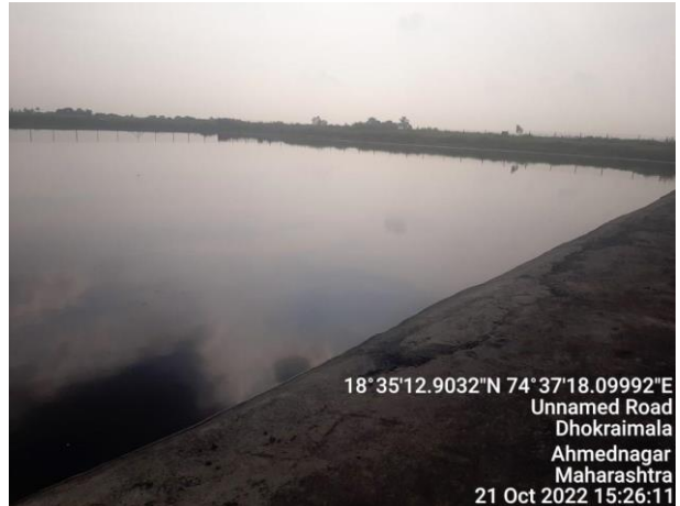
Photograph-8: 30 days lined spent wash storage lagoon.
