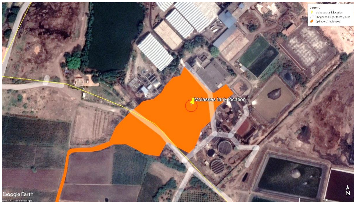
Figure 3.1: Image showing spillage of molasses inside factory premises
